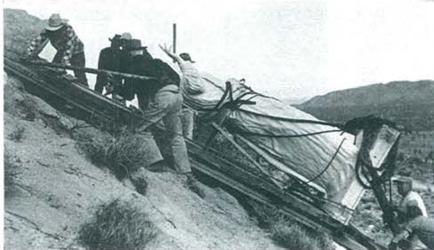
HALF WAY UP , statue inches along under combined efforts of men (above) and truck using pulley and cable. Wooden cradle was used to protect concrete.
